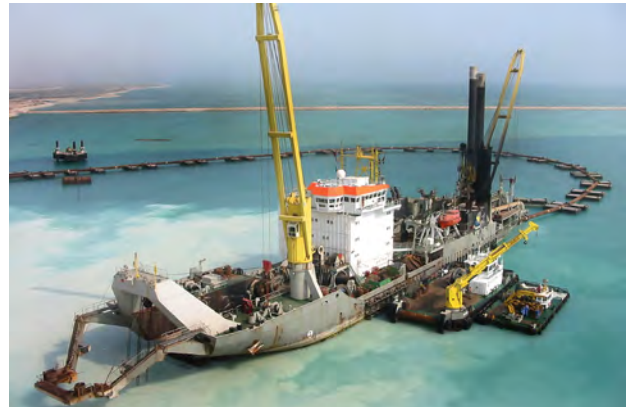
High accuracy positioning with no dependency on local shore based infrastructure for dredging
